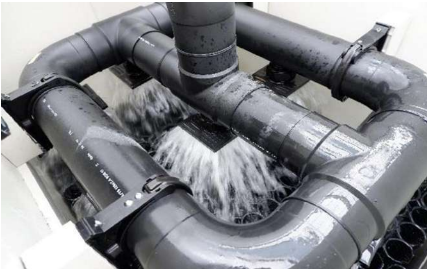
Figure 10. Top view of a CO 2 degasser
