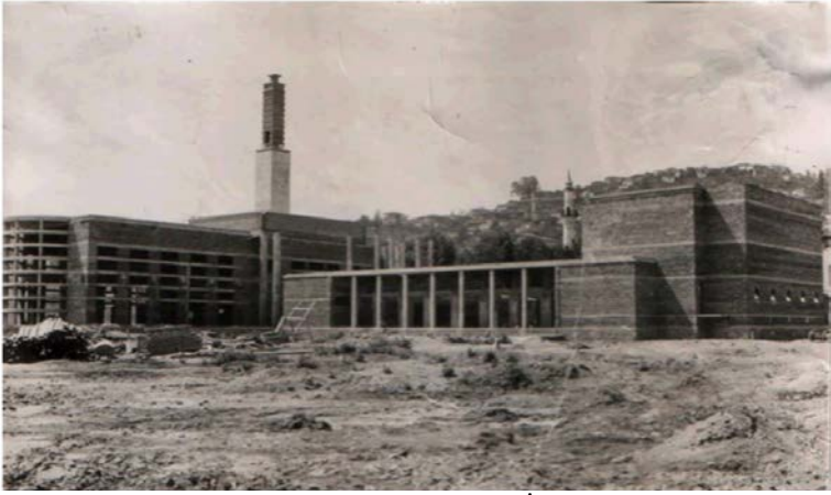
Construction of Izmit Community Center (İlker Kumral Archives)
