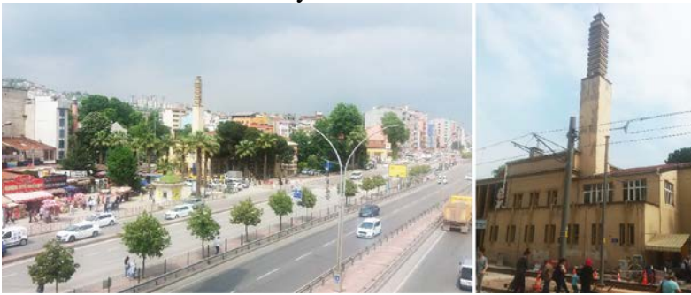
Izmit Community Center Present Position(İbrahim Türkeri Archive)
