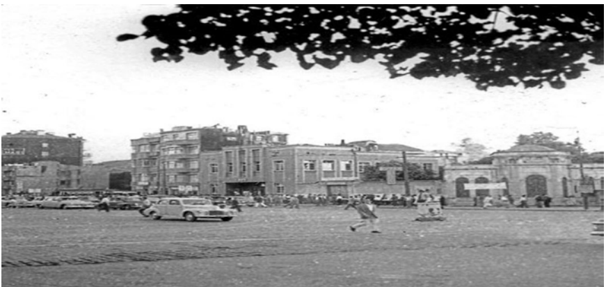
Figure 5. A Photography Construction Process of from Vatan Street(Sözcü Archive, 2016).
