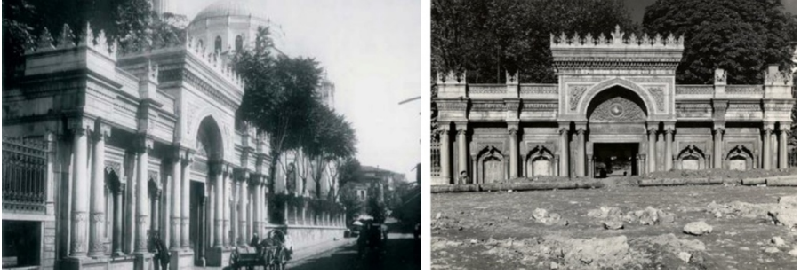
Figure9. The state of Pertevniyal Valide Sultan Mosque before and after road arrangements (İşli, 2008)
